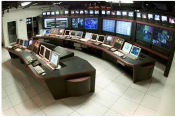
Gambar 5.23. Master Control Room di STV Bandung
